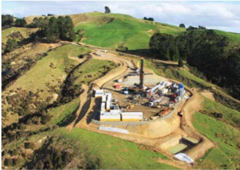
Figure 7: Ngapaeruru-1 exploratory well site (Source: TAG Oil)
