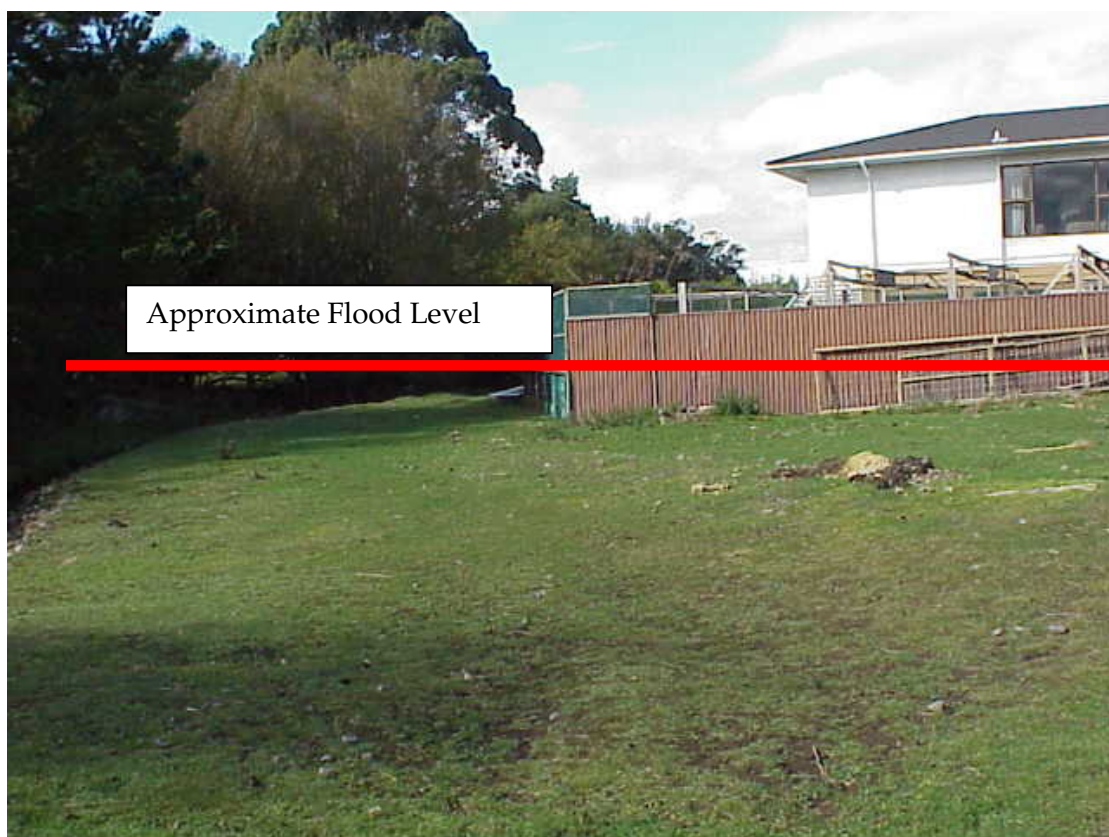
Figure 19: Approximate Flood Level at Jeffcoat House, Charlotte Street, Takapau
