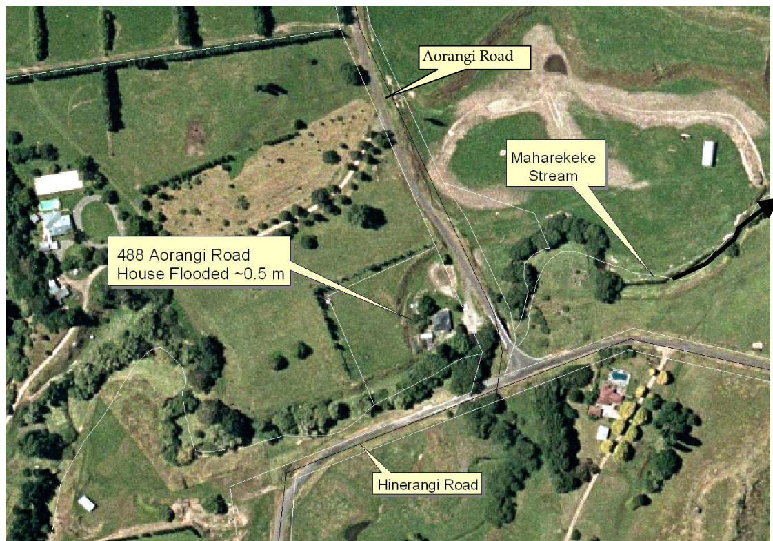
Figure 20: Flooding from Maharakeke Stream, Aorangi Road.
