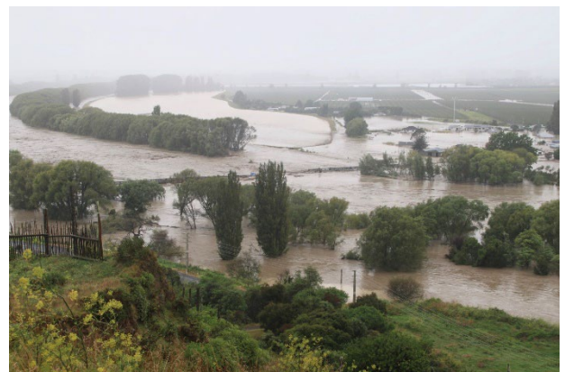
Figure 4: Redcliffe Bridge at Taradale, Tūtaekurī River
