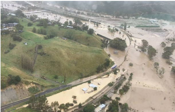
Figure 2: Eskdale SH5/SH2 Intersection; Esk River in flood, Cyclone Gabrielle
