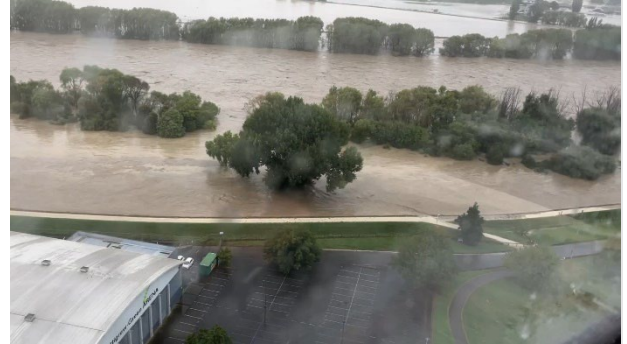
Figure 3: Taradale IRG upgraded stopbank, 14 February 2023
