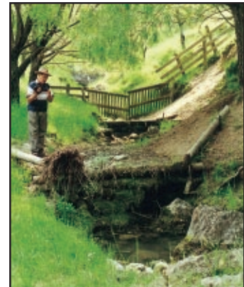
Two 15 year old rail & netting dams effectively stopping any gully deepening.
