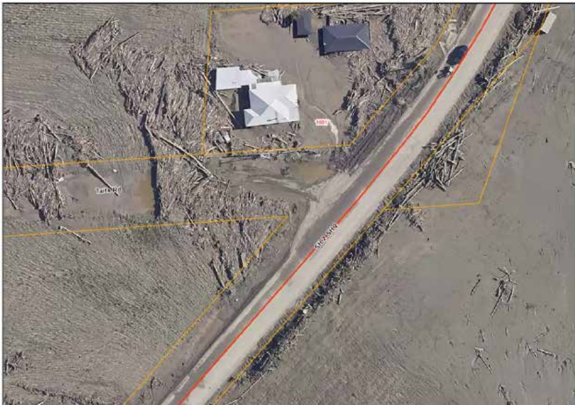
Figure 13.1 - Woody Debris build-up near Esk River mouth.
