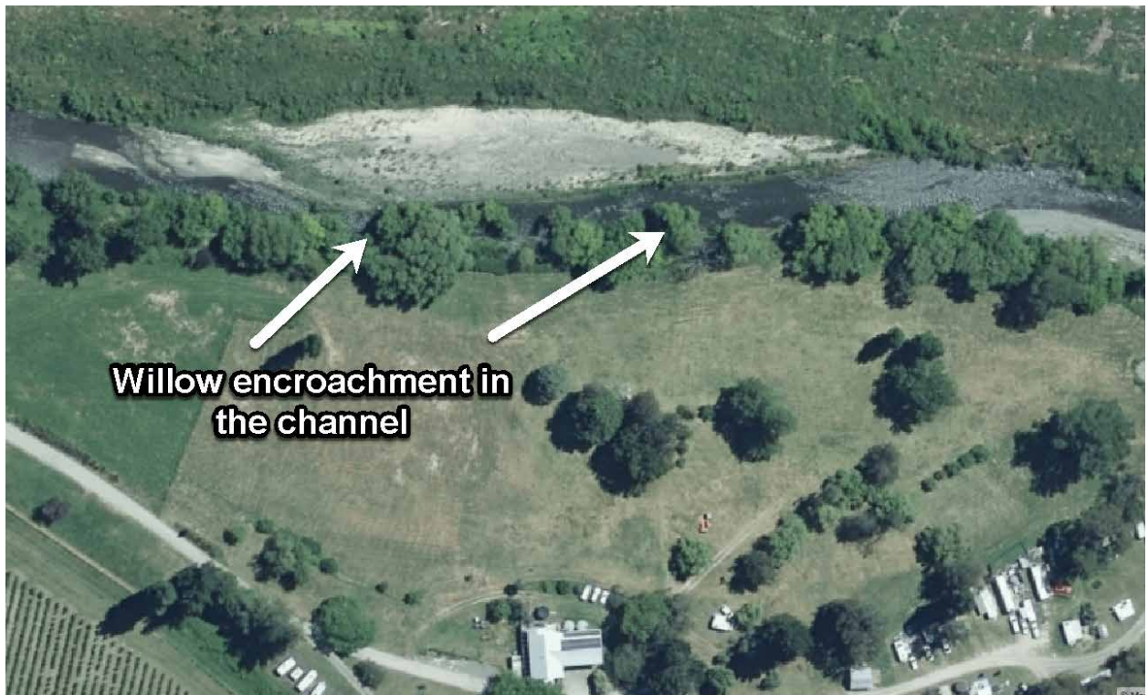
Figure E3 Willow Encroachment into Esk River
