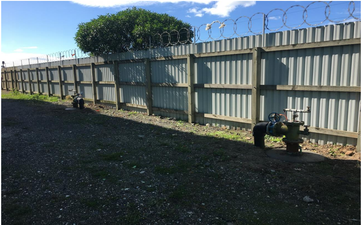
Photo taken approximately 10m away showing bore and surrounding area
