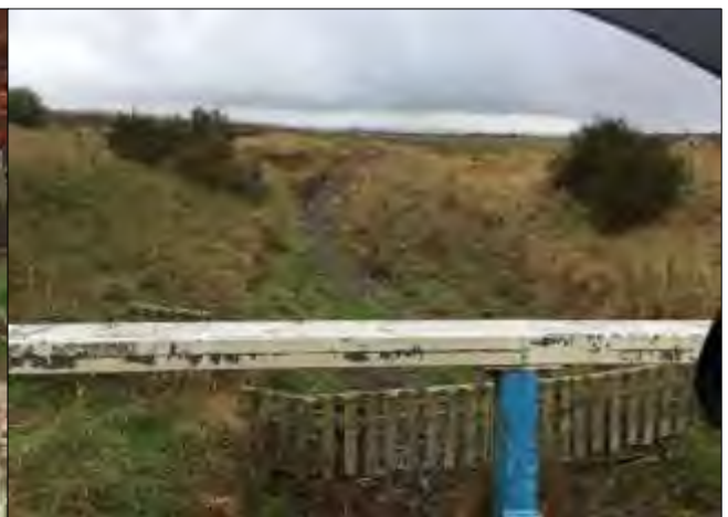
Figure 20. Chestermans Bridge. Ongaonga (view NW).
