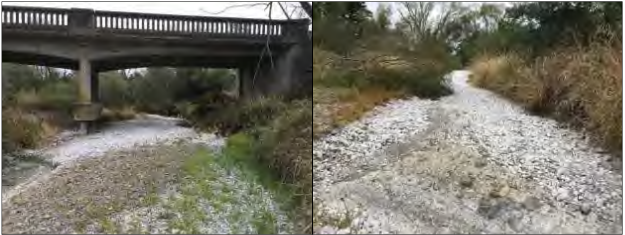
Figure 7. Mangamauku Stream, SH50, Tikokino (L = view west; R = view east). No surface water observed.
