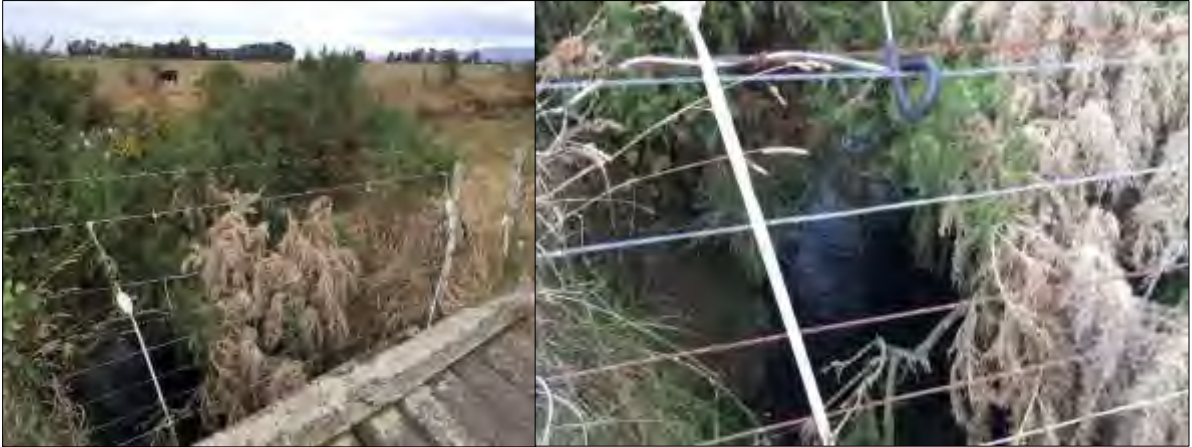
Figure 11. Kahahakuri Stream gaining reach, Swamp Road, Ongaonga.
