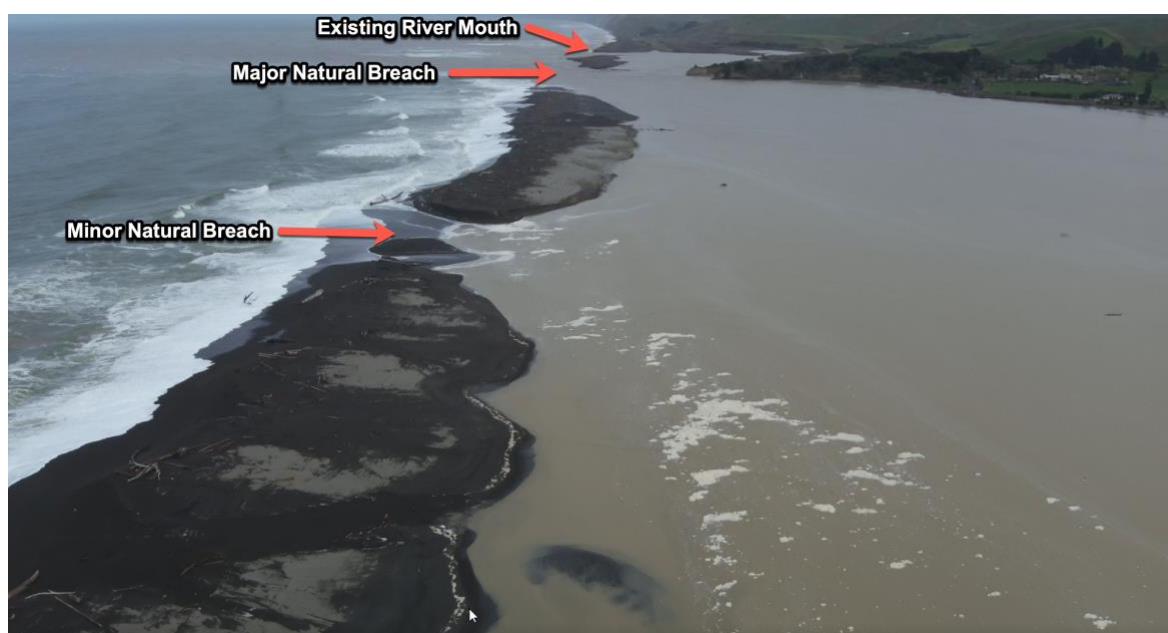
Figure 4-5 Aerial image showing the existing river mouth and natural breaches that occurred during the event (Source FENZ UAV)
