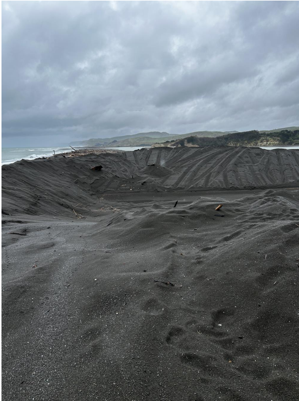
Figure 4-3 Wairoa River bar seaward coffer dam and upstream pilot channel (9 August 2024)
