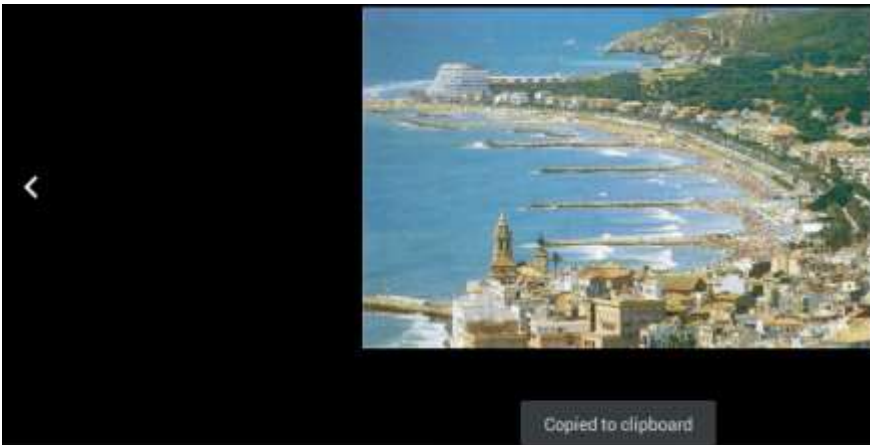
Groynes in Sitges, Catalonia, Spain
