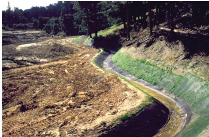
Waterway Diversion on a Highway Project
