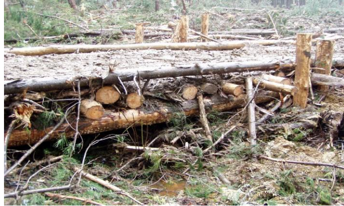
Bridge on a Forestry Project Constructed of Available Wood
