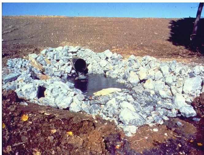
Rock Outlet Protection for a Temporary Drain
