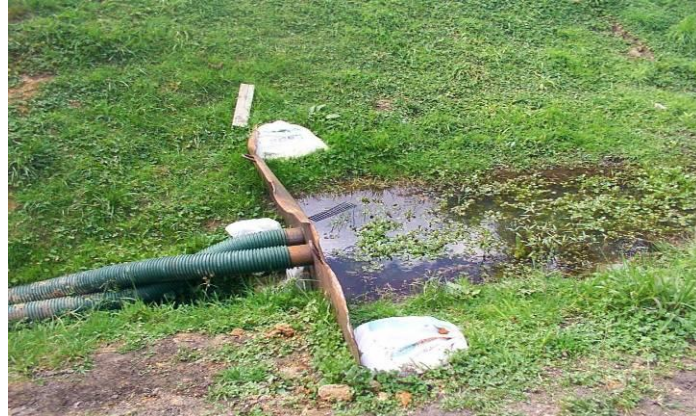
Water Being Diverted Past a Construction Site
