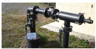
3. Meter too close to tee, obstruction directly up stream of meter and insufficient straight length of pipe.
