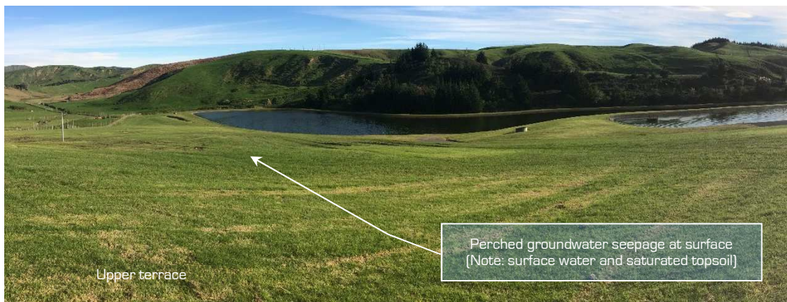
Figure 6: Panoramic view north over site [Note: Perched groundwater seepage at surface].
