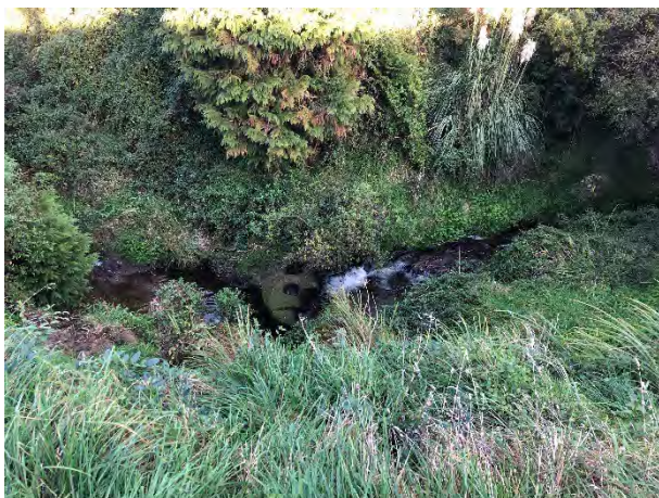
Plate 3-33: Pohatanui Stream channel
