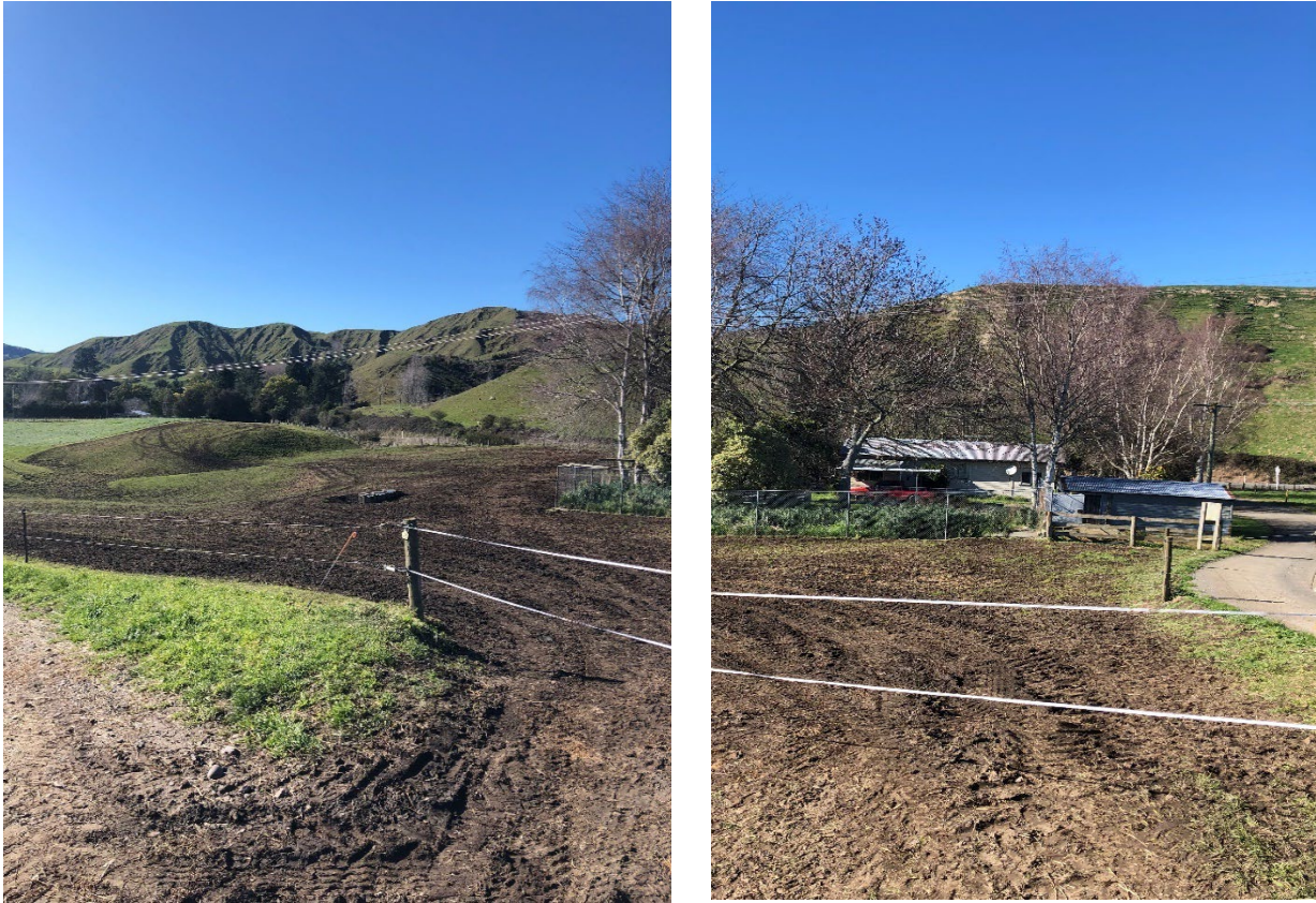
Figure 5: Site at southern end of the realignment
