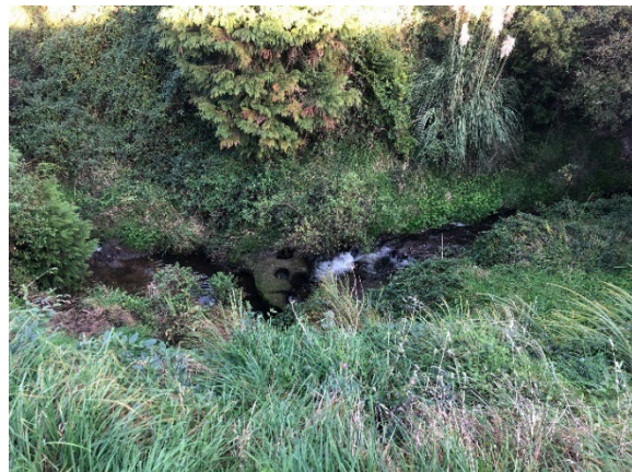
Figure 17: Kings Creek stream channel
