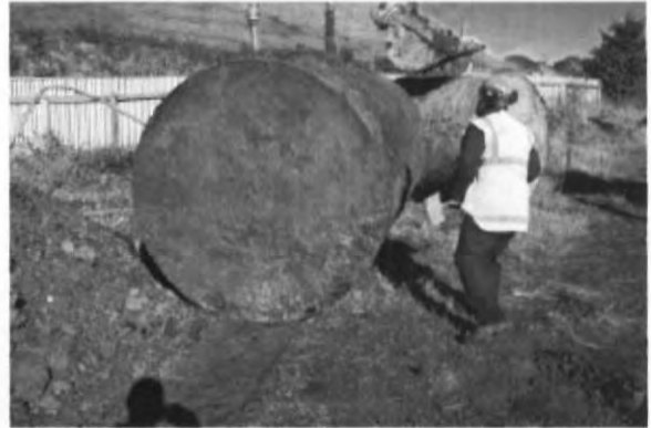
Tank 2 pit (with slight diesel residue on removal)
