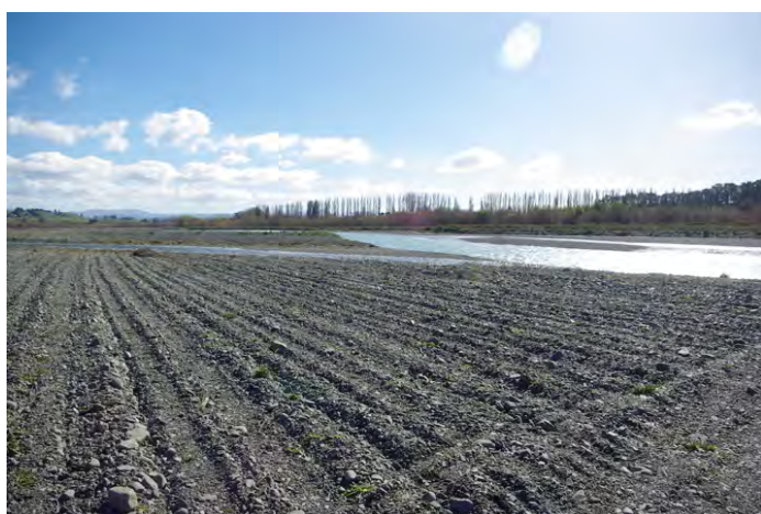
Figure 8. Example of a Hawke's Bay braided riverbed having recently been beach raked.
