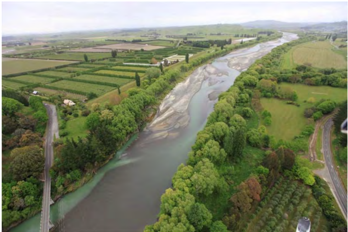
Figure 4: Typical section of braided Tutaekuri River channel (looking up-river of Puketapu Road bridge). Note stopbank on the far side of the river
