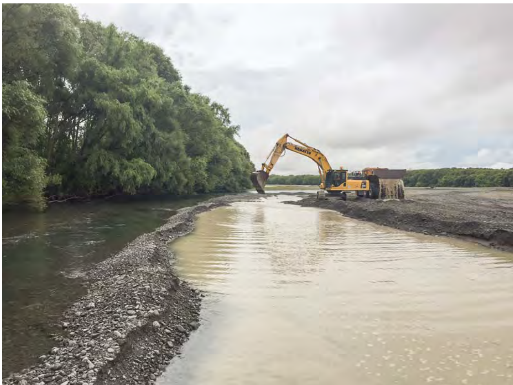
Figure 14: Typical gravel extraction operations showing works bunded from main river on far left (adjacent to willow trees).
