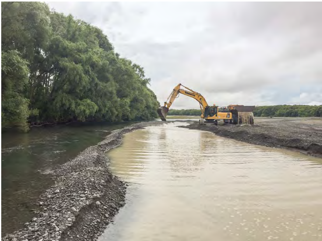
Figure 14: Typical gravel extraction operations showing works bunded from main river on far left (adjacent to willow trees).
