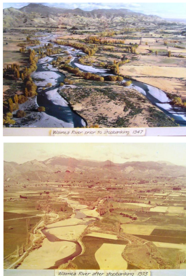
Figure 3. The Waimea River (Tasman District) before (upper) and after (lower) stop-banks were instated showing the simplification of channel form after flood protection infrastructure.
