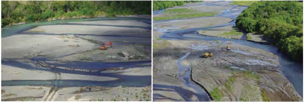
Figure 13: Typical gravel extraction operations
