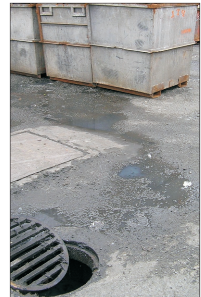
Ongoing contaminated runoff discharging to stormwater as a result of poor housekeeping
