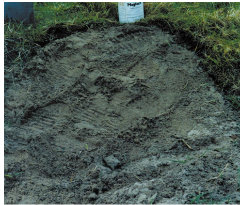
End result- burrow well sealed and backfilled
