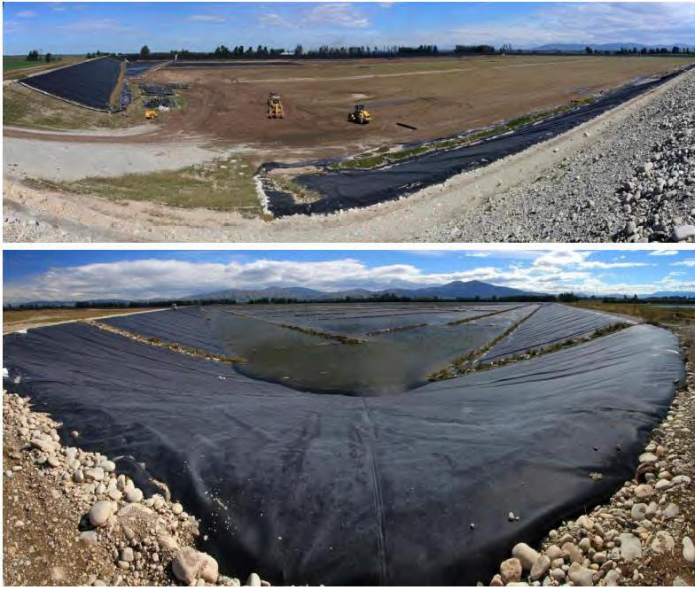
Figure 4: Mayfield Hinds Irrigation – Carew Pond lining.
