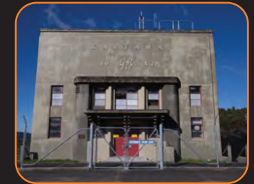
KAITAWA POWER STATION (36 MW)
