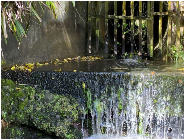
Figure 3-10 Outlet at cross-culvert C12200 with a large drop.
