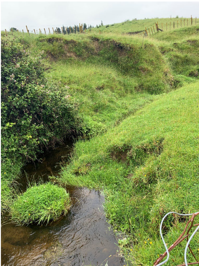
Figure 4-1 Steep embankments and watercourses, such as the above at chainage 13190 will require protection as works proceed.
