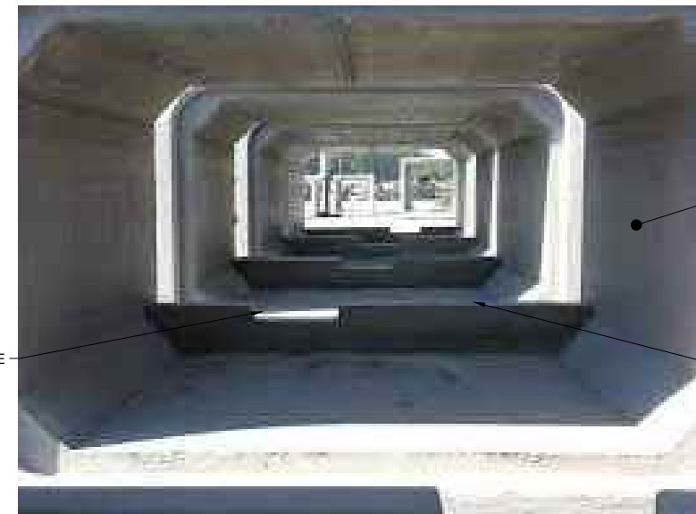
PRECAST BOX CULVERT WITH FISH PASSAGE NTS
