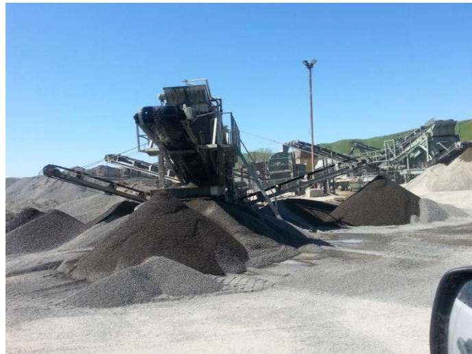
Figure 3: Ngaruroro River gravel being processed
