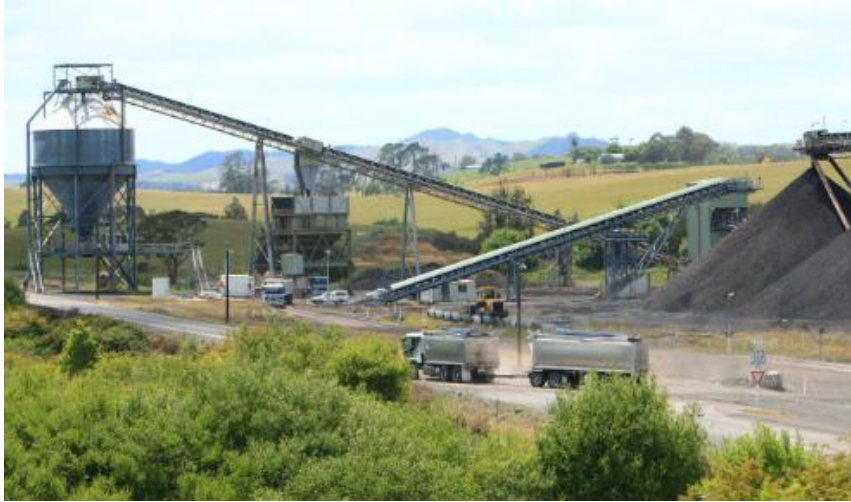
Figure 17: Photograph of coal load out area at Solid Energy's Rotowaro mine in Waikato.
